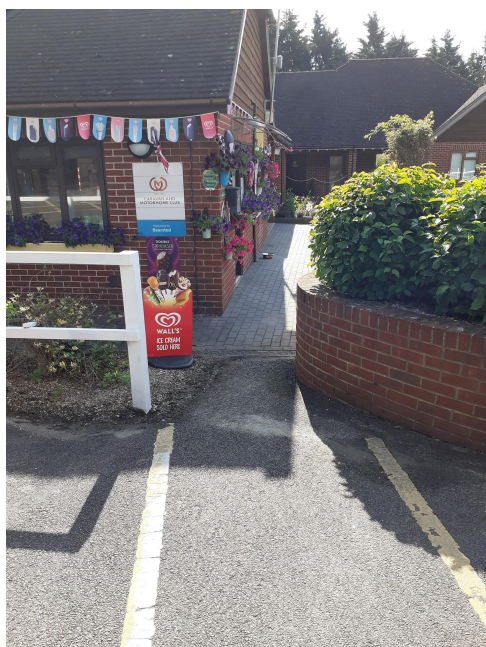
Building housing Toilet Facilities, as well as reception
