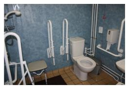
controlled shower has the control at 900mm height, and a hand shower adjustable from 1300mm to 1900mm height. The shower has a drop-down seat, as well as a loose shower chair and fixed vertical and horizontal grab rails.
