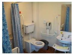
floor. The shower does not have a low-level shelf and the sliding rail attachment is too high to reach from a seated position. Grab rails are lacking in colour and contrast.
