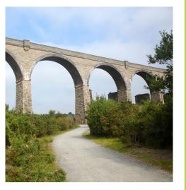
Interesting fact...the present nine-arch stonework viaduct replaces an earlier structure designed in 1863 which was made up of a timber deck and supported by timber trestles springing from eleven masonry piers.
