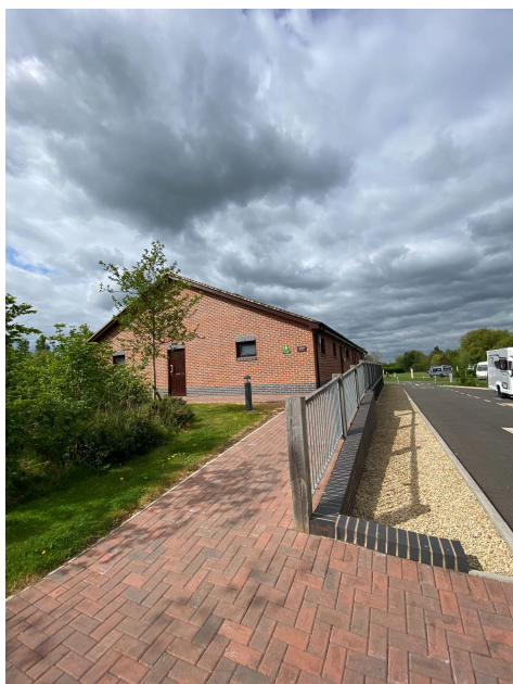
Ramp to Toilet Block
