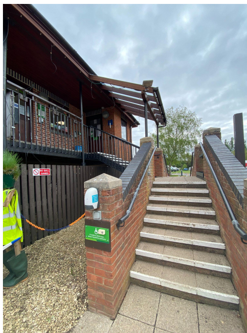
Stairs to reception
