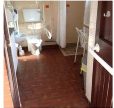
The shower area is 800mm square, with curtain around, thermostatically controlled shower with controls at 900mm height, and shower head adjustable from 750mm to 1500mm height. The shower has a drop-down seat, and fixed vertical and horizontal grab rails. The turning circle for a wheelchair user is restricted to 1100mm by the baby changing worktop.
